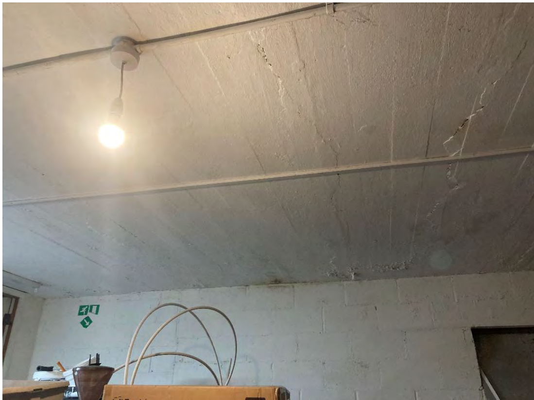
Photograph 28: Condition inside Arches No. 146 – 147. Widespread cracking.
