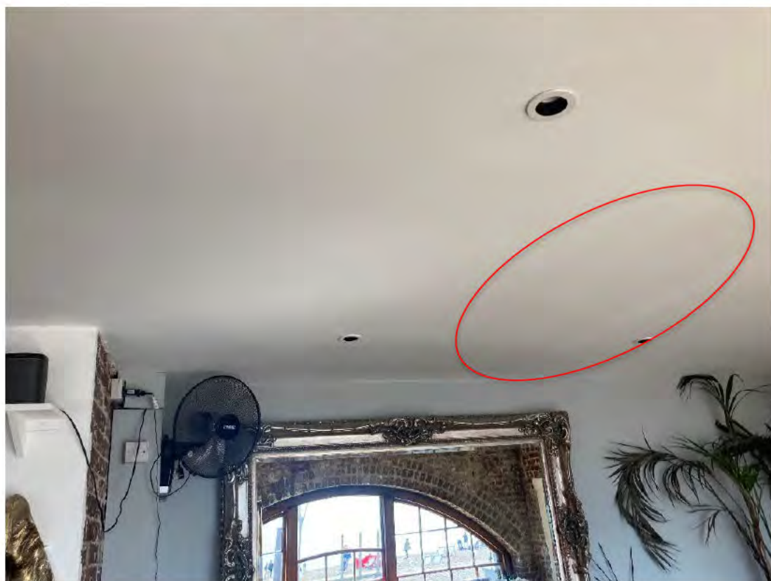
Photograph 23: General condition inside Arches No. 142 – 144. Recently painted, widespread water staining is still evident.
