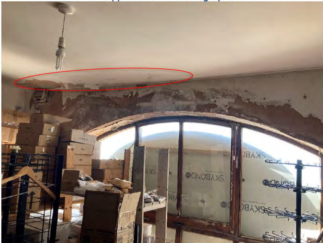
Photograph 2: General condition inside Arch No. 125. Note paint flaking and water staining along façade edge.
