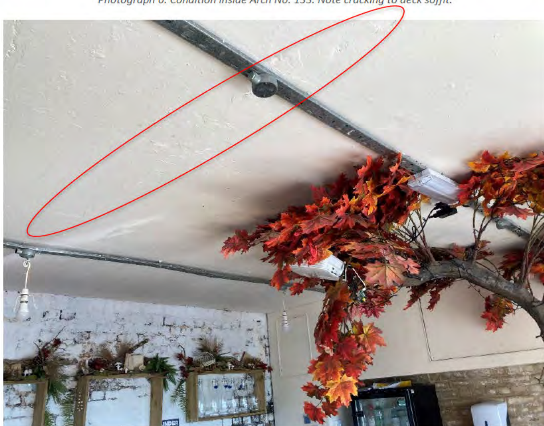
Photograph 7: Condition inside Arch No. 133. Cracking to deck soffit extends throughout the entire unit.
