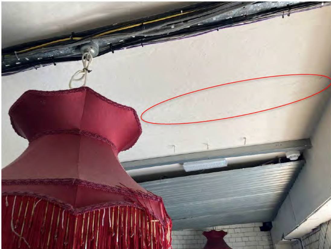
Photograph 8: Condition inside Arch No. 134. Note cracking to deck soffit.
