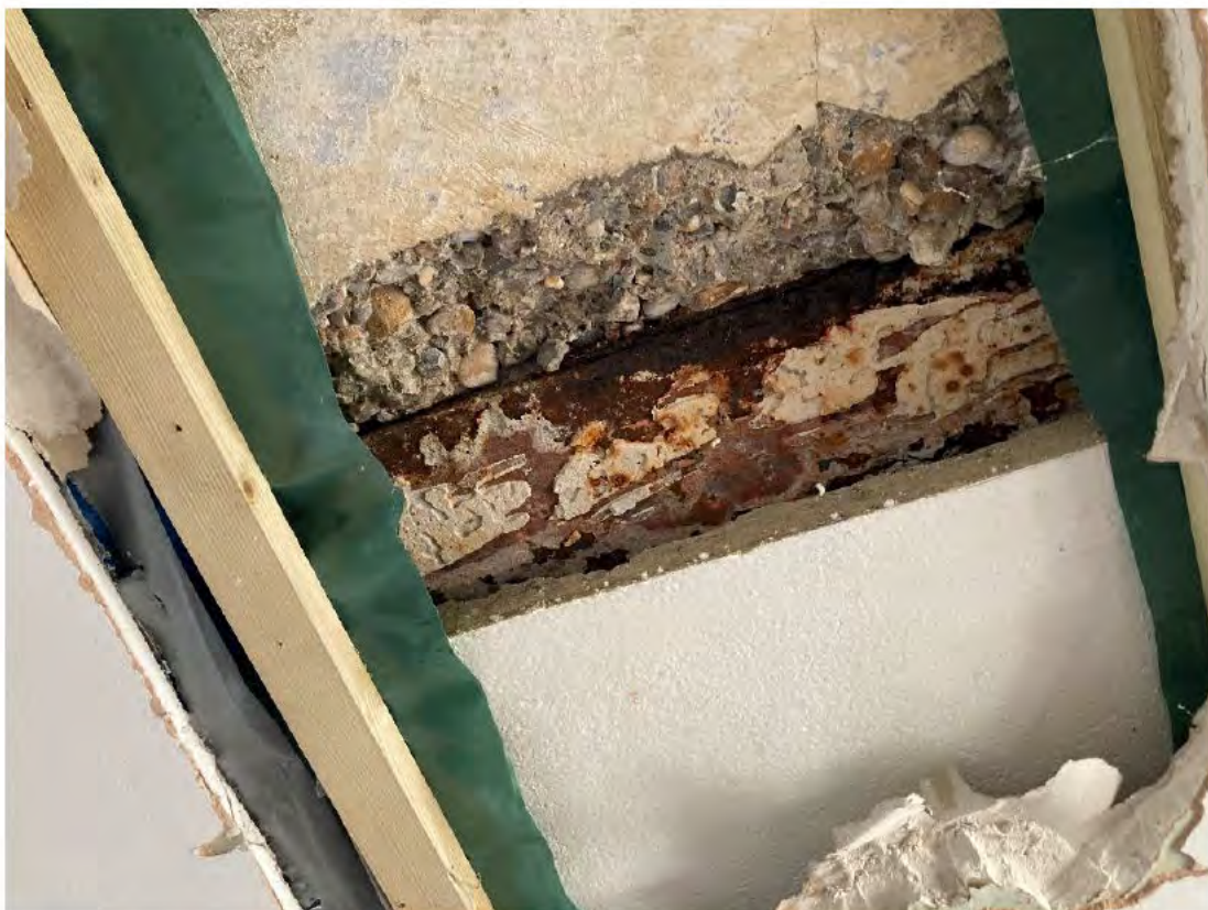
Photograph 3: Arch No. 125. Deck soffit presents honeycombing and corrosion to steel joist.
