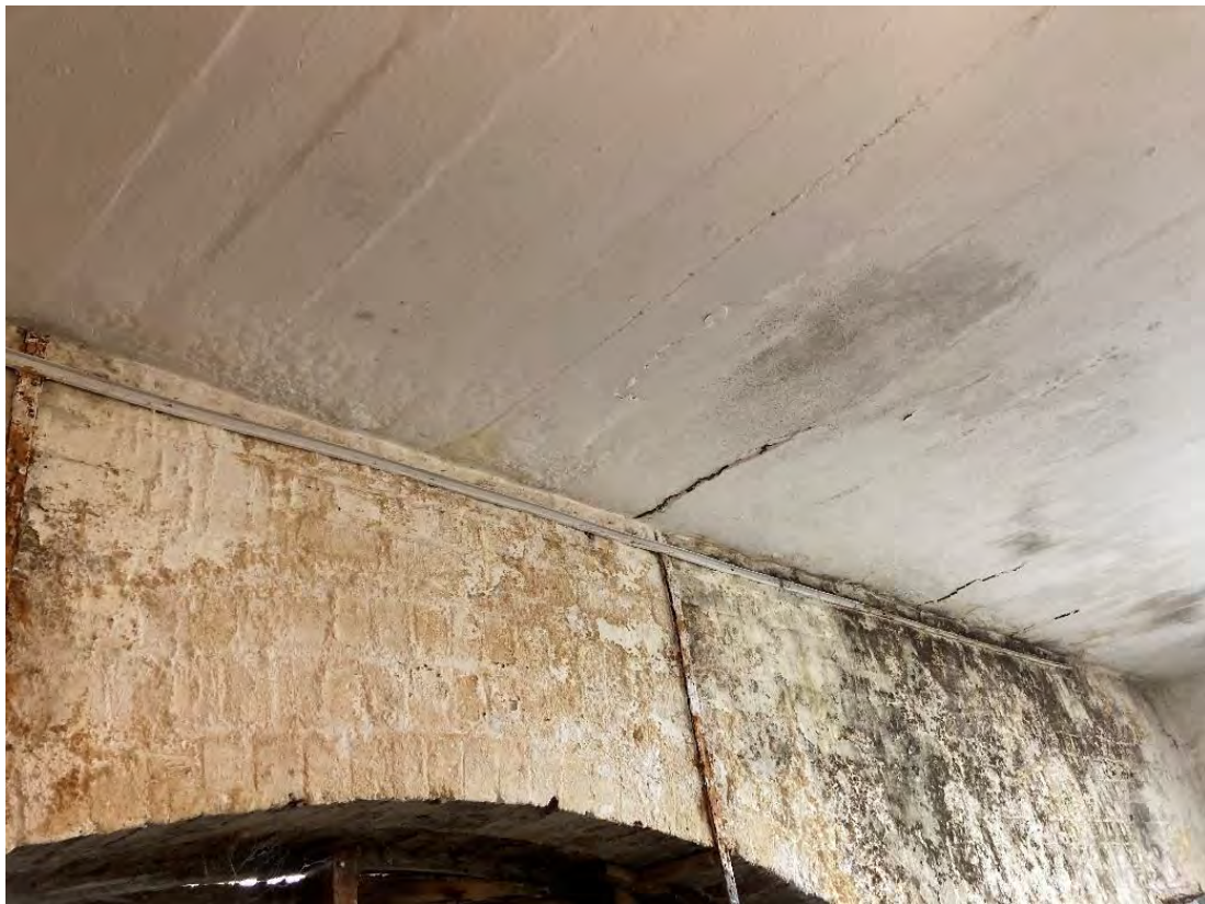
Photograph 27: Condition inside Arches No. 146 – 147. Significant cracking and water seepage.
