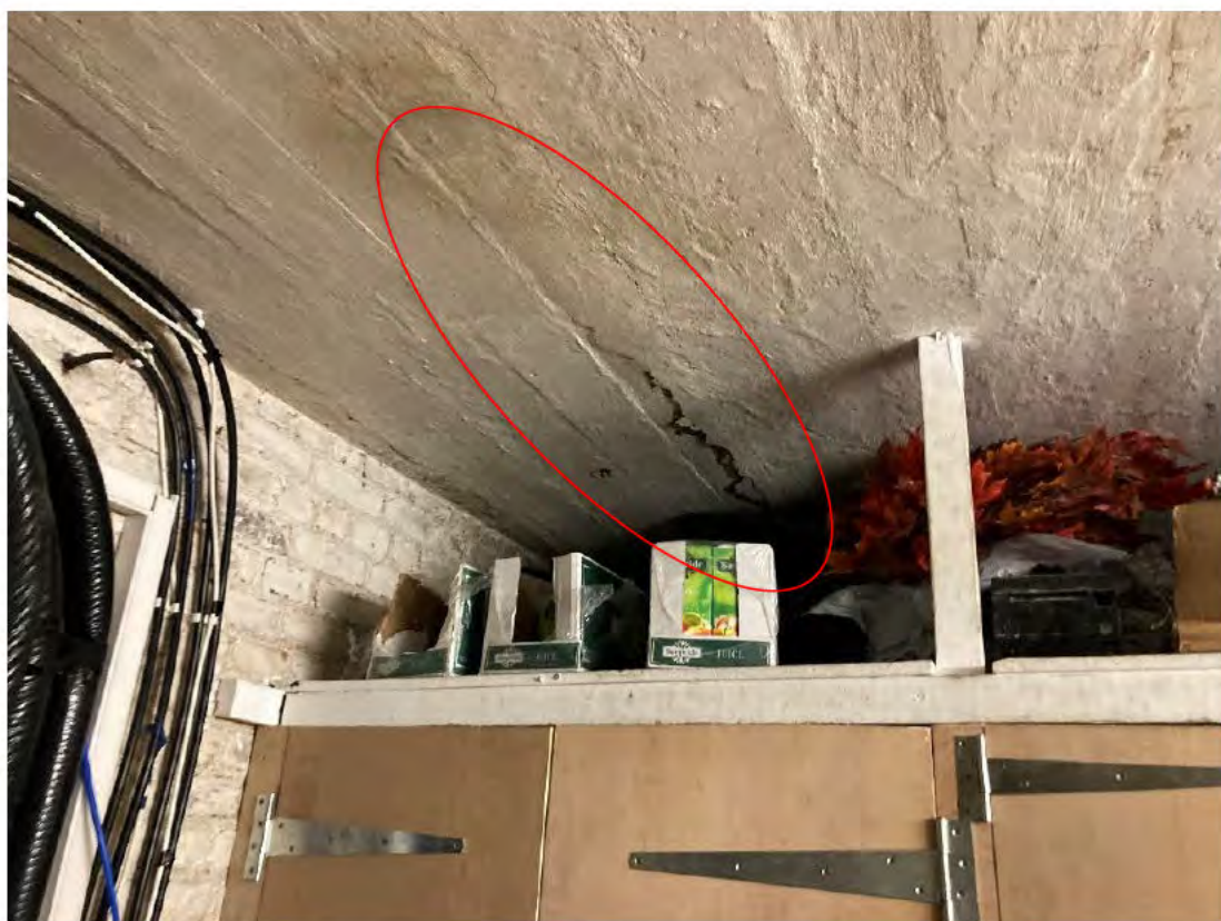
Photograph 13: Condition inside Arch No. 135. Note significant crack and water staining and seepage to deck soffit.
