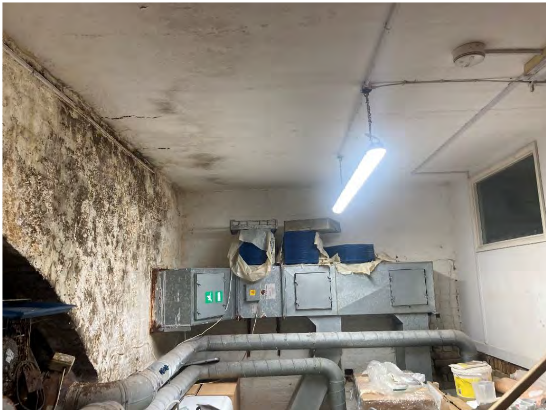
Photograph 26: General condition inside Arches No. 146 – 147 presenting widespread water staining and seepage.
