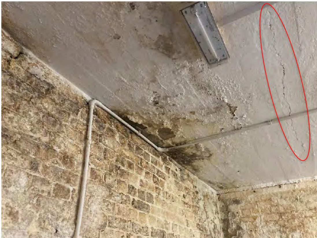
Photograph 30: Condition inside Arches No. 146 – 147. Isolated area of paint flaking and water seepage and staining. Note significant crack too.
