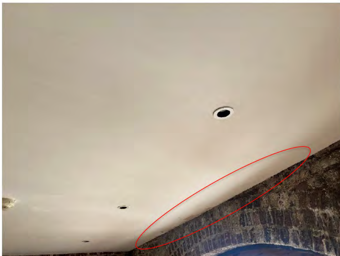
Photograph 24: General condition inside Arches No. 142 – 144. Note paint flaking and water staining along façade edge.
