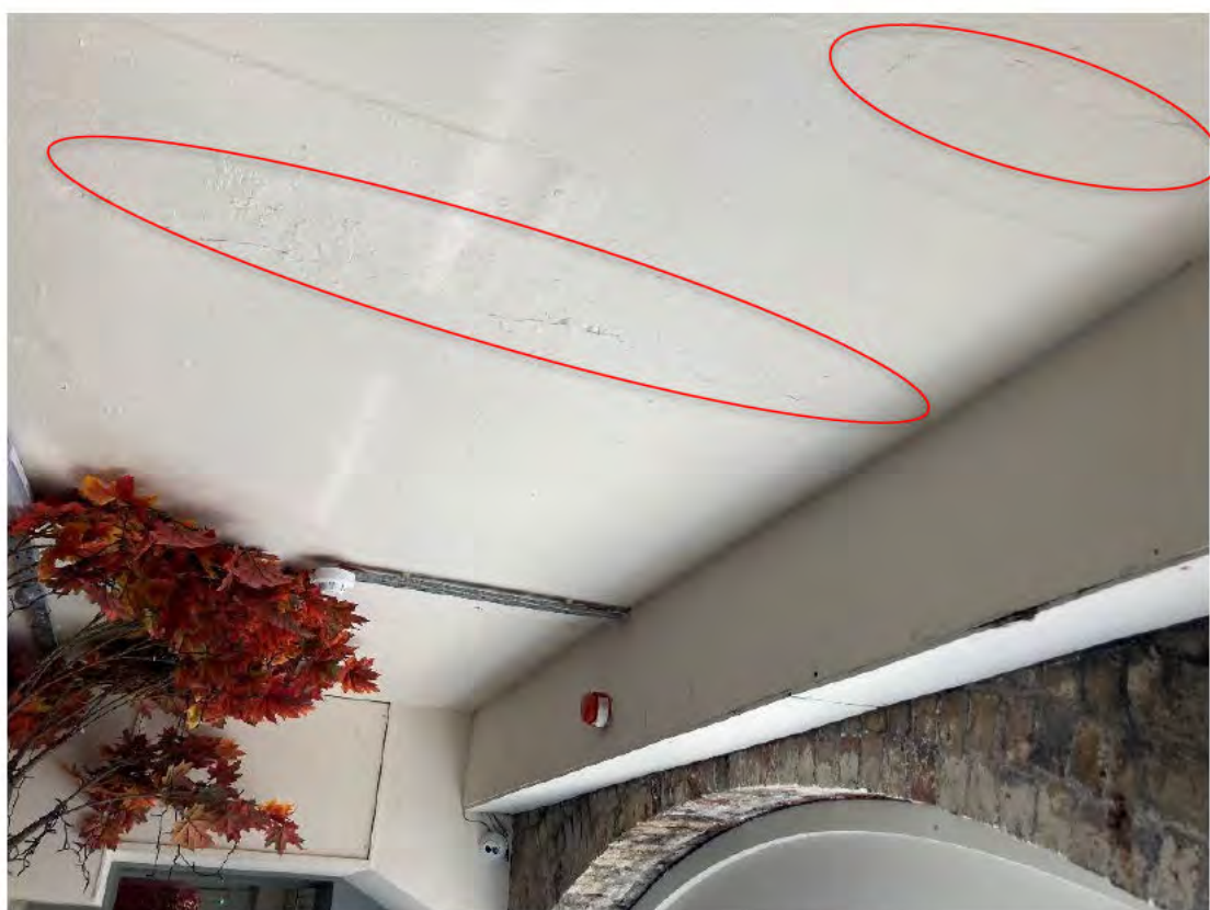
Photograph 6: Condition inside Arch No. 133. Note cracking to deck soffit.
