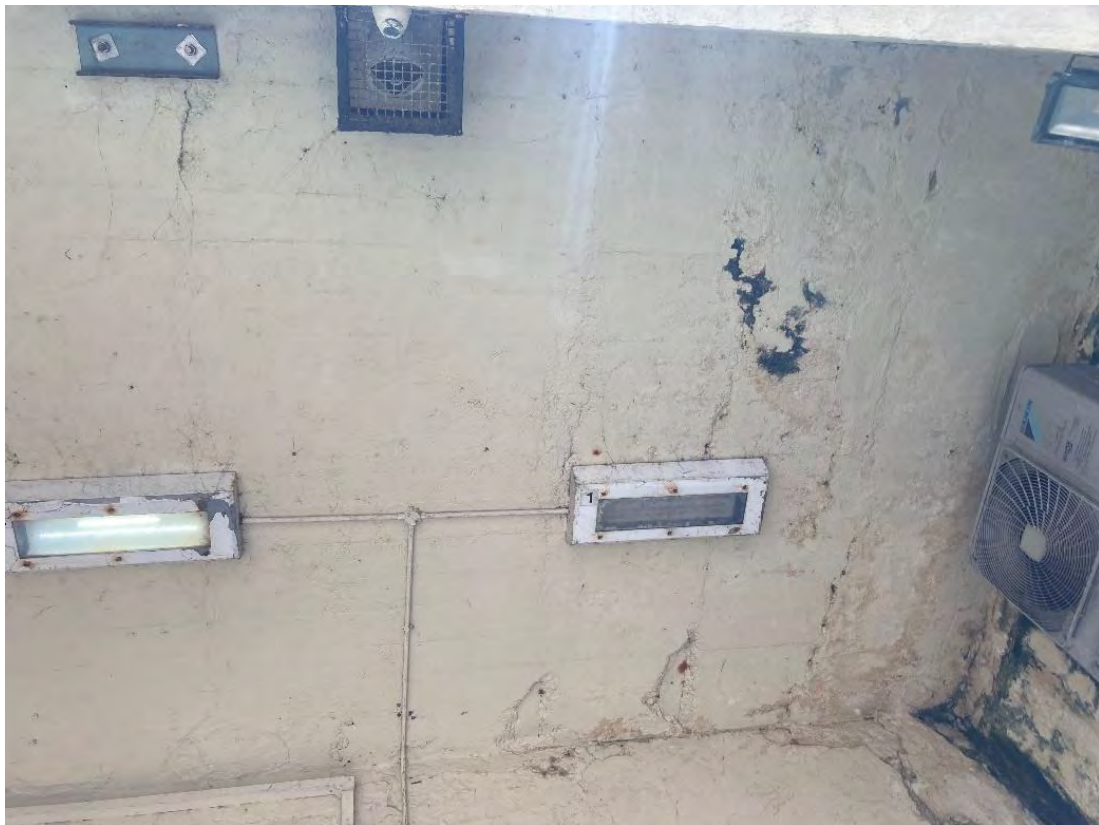
Photograph 33: General condition inside Arch No. 149 presenting significant cracks and areas of water staining and seepage.
