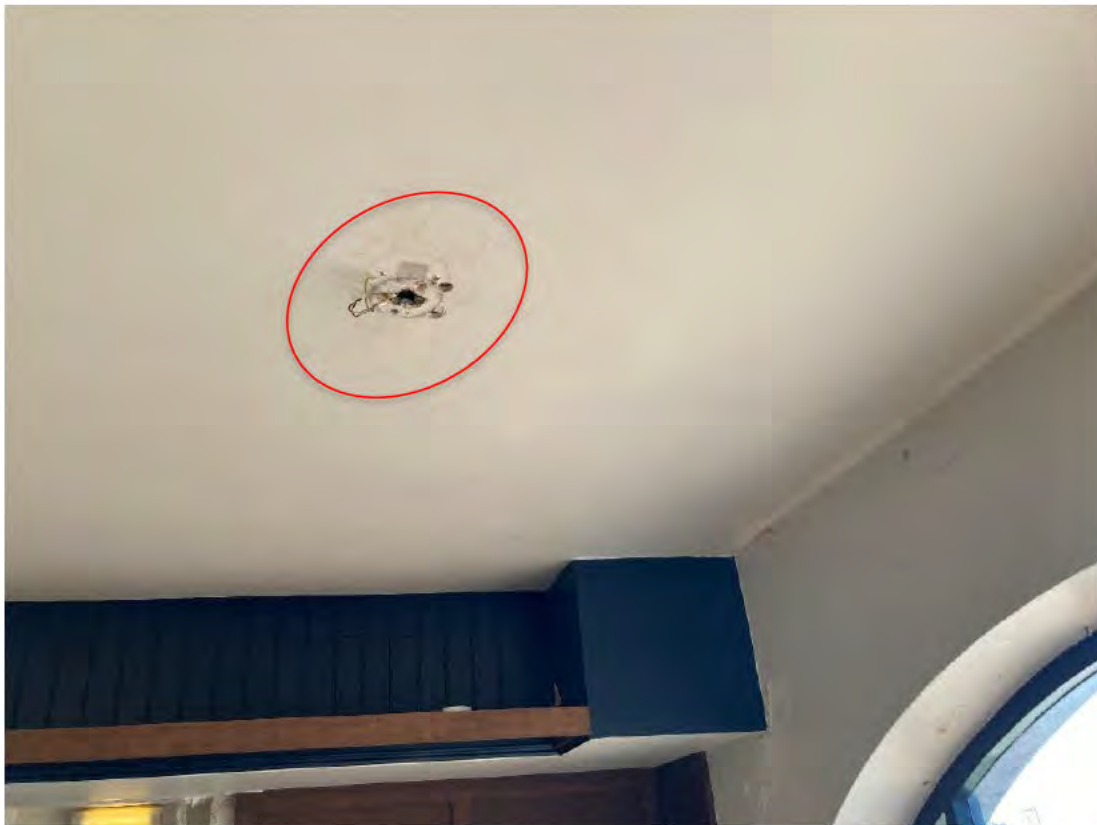
Photograph 18: General condition inside Arch No. 139. Recently painted, however surface defects to concrete deck around electric ducting openings noted.
