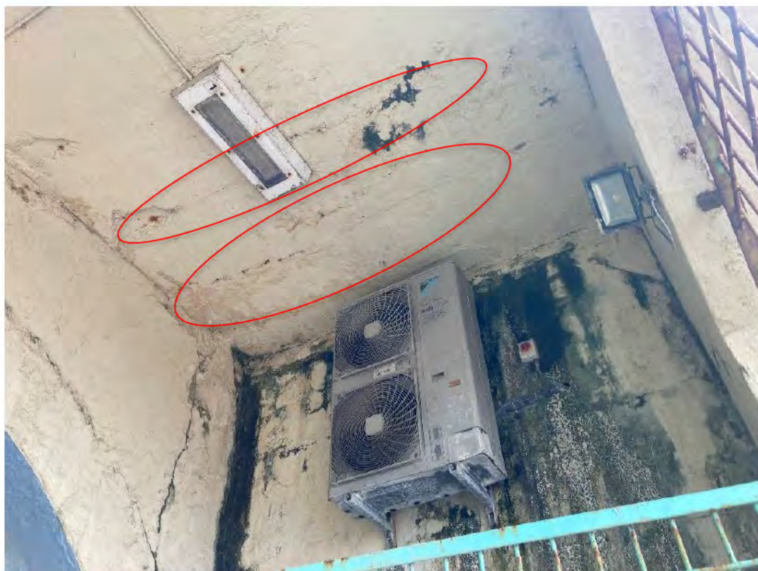
Photograph 34: Condition inside Arch No. 149 Note evidence of abundant water seepage through deck joint. Also note presence of significant cracks and spalls.
