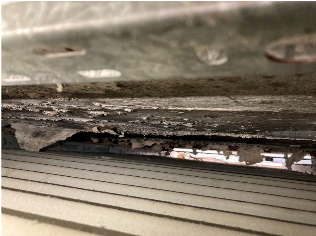
Photograph 10: Arch No. 134. Deck soffit presents paint flaking above ceiling panel. Access too constrained to identify associated deterioration, however evidence of water dripping is noted in previous photograph.
