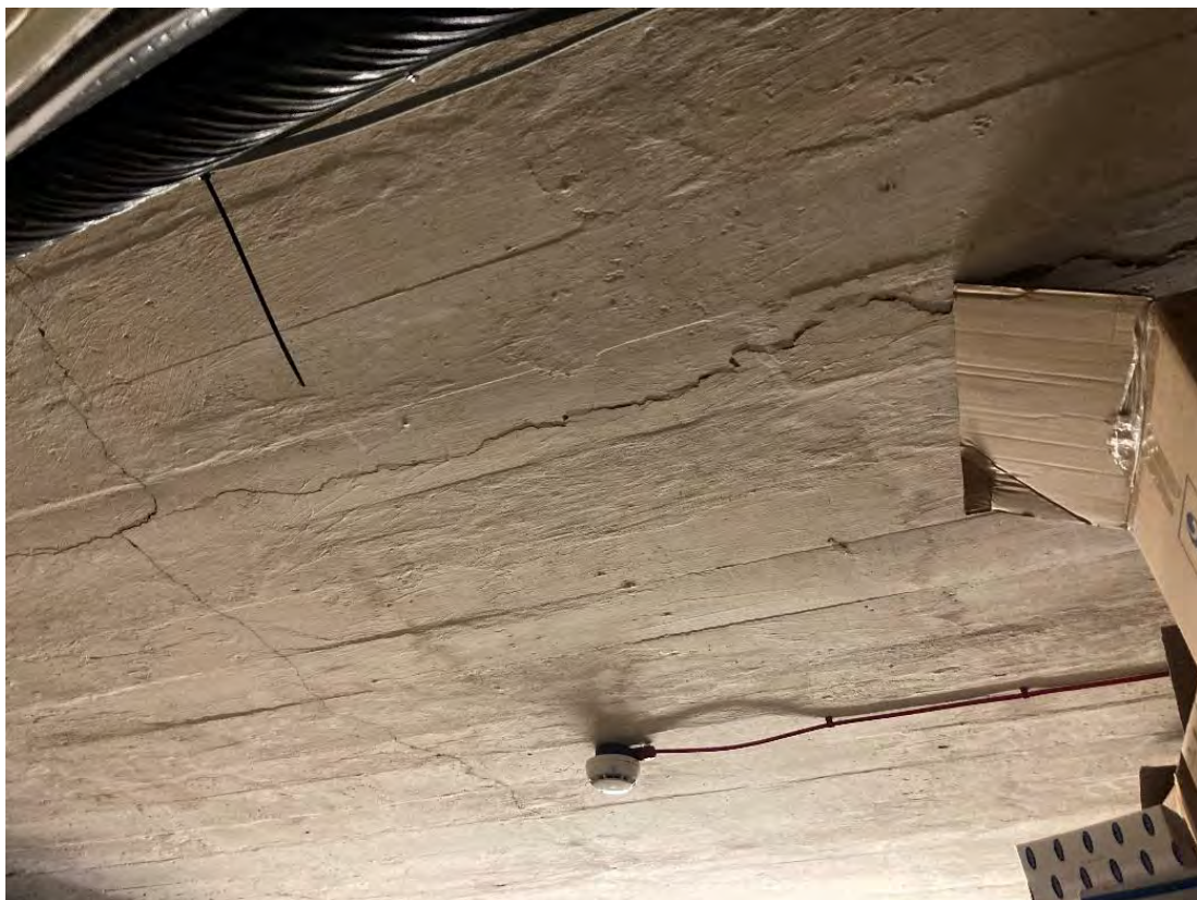
Photograph 11: Condition inside Arch No. 135. Deck soffit presents widespread cracking.
