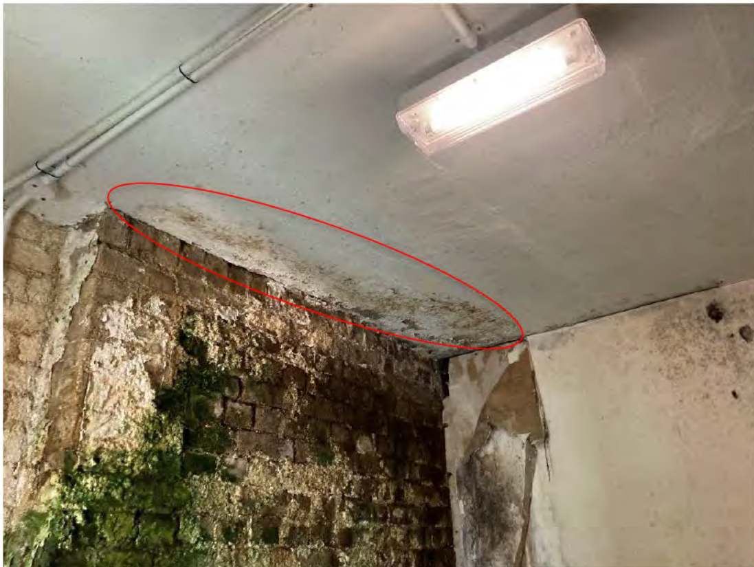
Photograph 20: General condition inside Arch No. 140. Note paint flaking and water staining and seepage.
