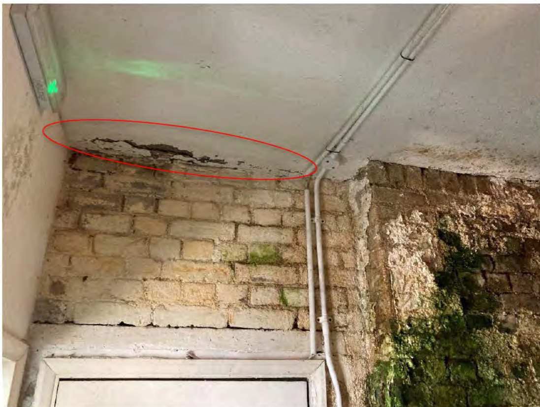
Photograph 19: General condition inside Arch No. 140. Note paint flaking, significant cracking, water staining and seepage.
