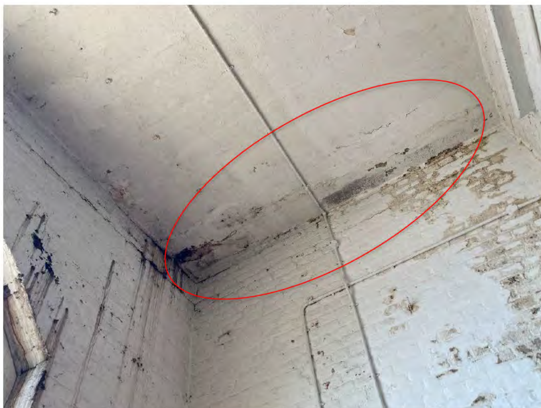
Photograph 17: General condition inside Arch No. 138. Note paint flaking, significant cracking, water staining and seepage.
