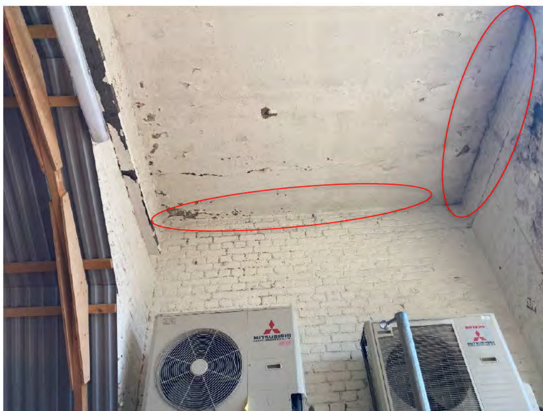
Photograph 16: General condition inside Arch No. 138. Note paint flaking, significant cracking, water staining and seepage.
