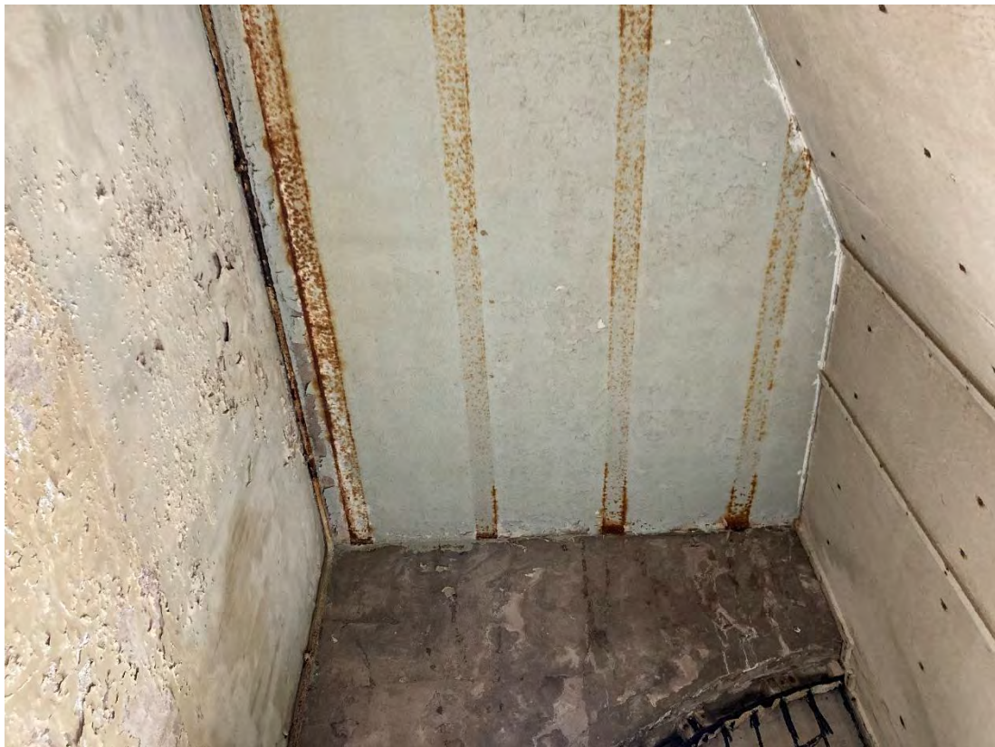
Photograph 32: General condition inside Arch No. 148b showing extensive corrosion to the filler joists.
