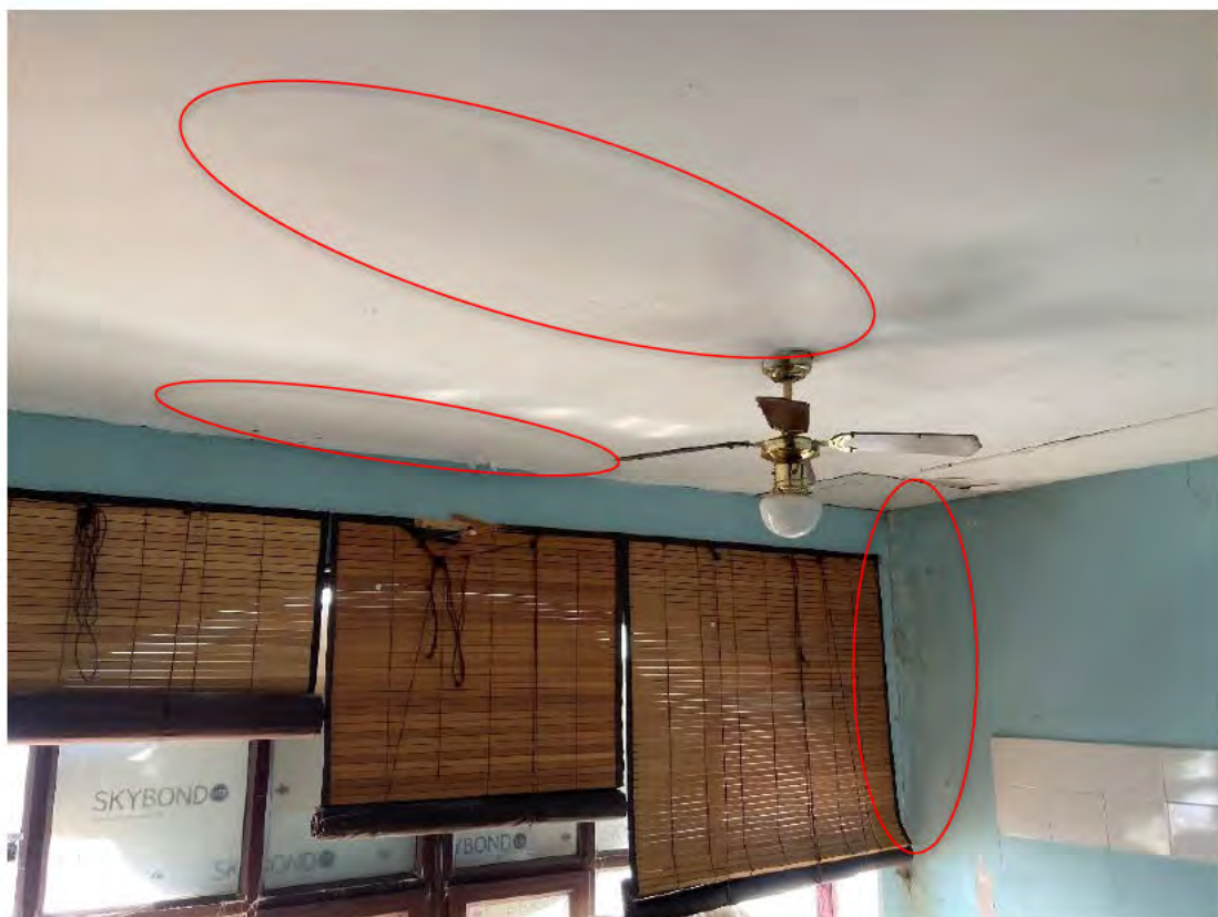
Photograph 4: General condition inside Arch No. 126. Note paint flaking and water staining painted over.
