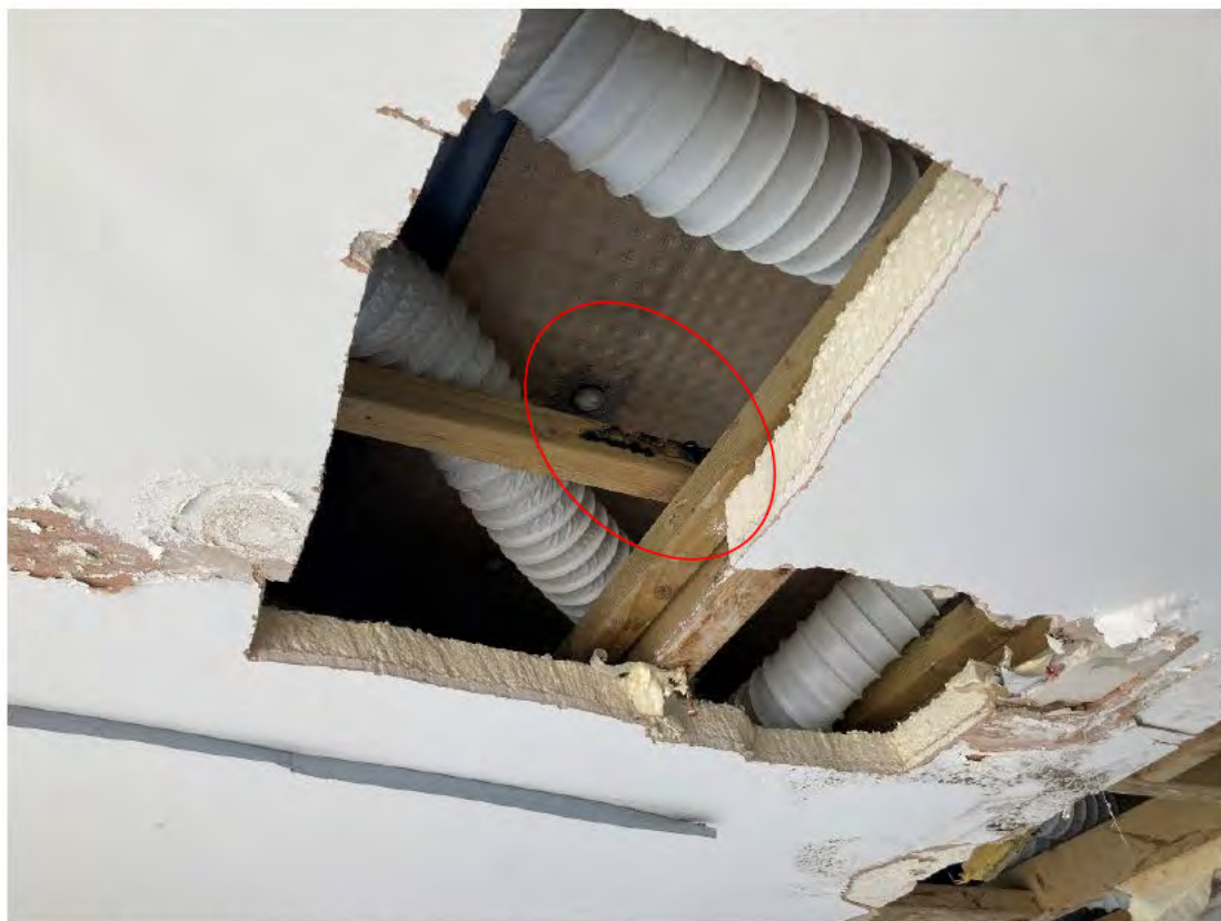
Photograph 15: Arch No. 137 is clad. Timber purlins supporting cladding present localised water staining and decay.
