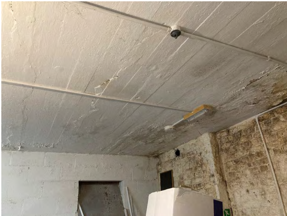
Photograph 29: Condition inside Arches No. 146 – 147. Widespread cracking.
