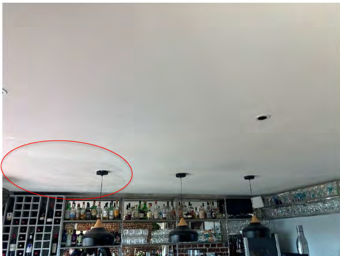
Photograph 22: General condition inside Arches No. 142 – 144. Recently painted, widespread water staining is still evident.
