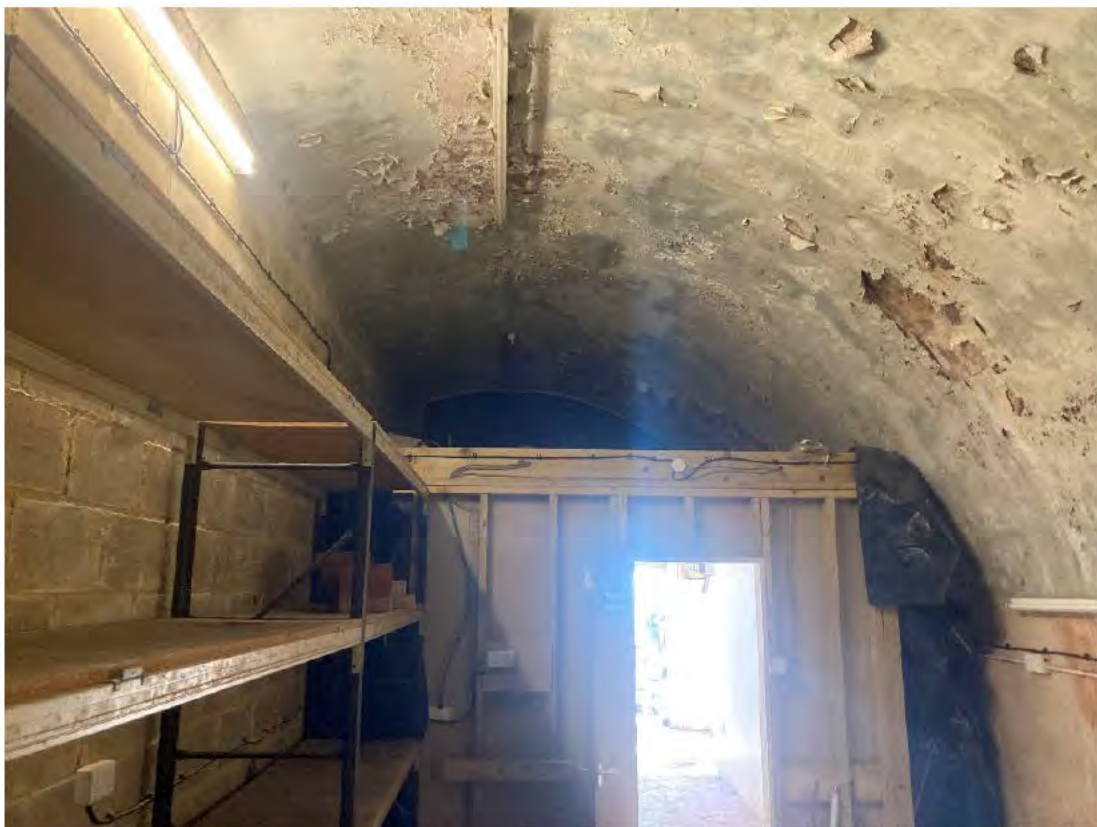
Photograph 31: General condition inside Arch No. 148a (masonry arch) presenting widespread paint flaking.
