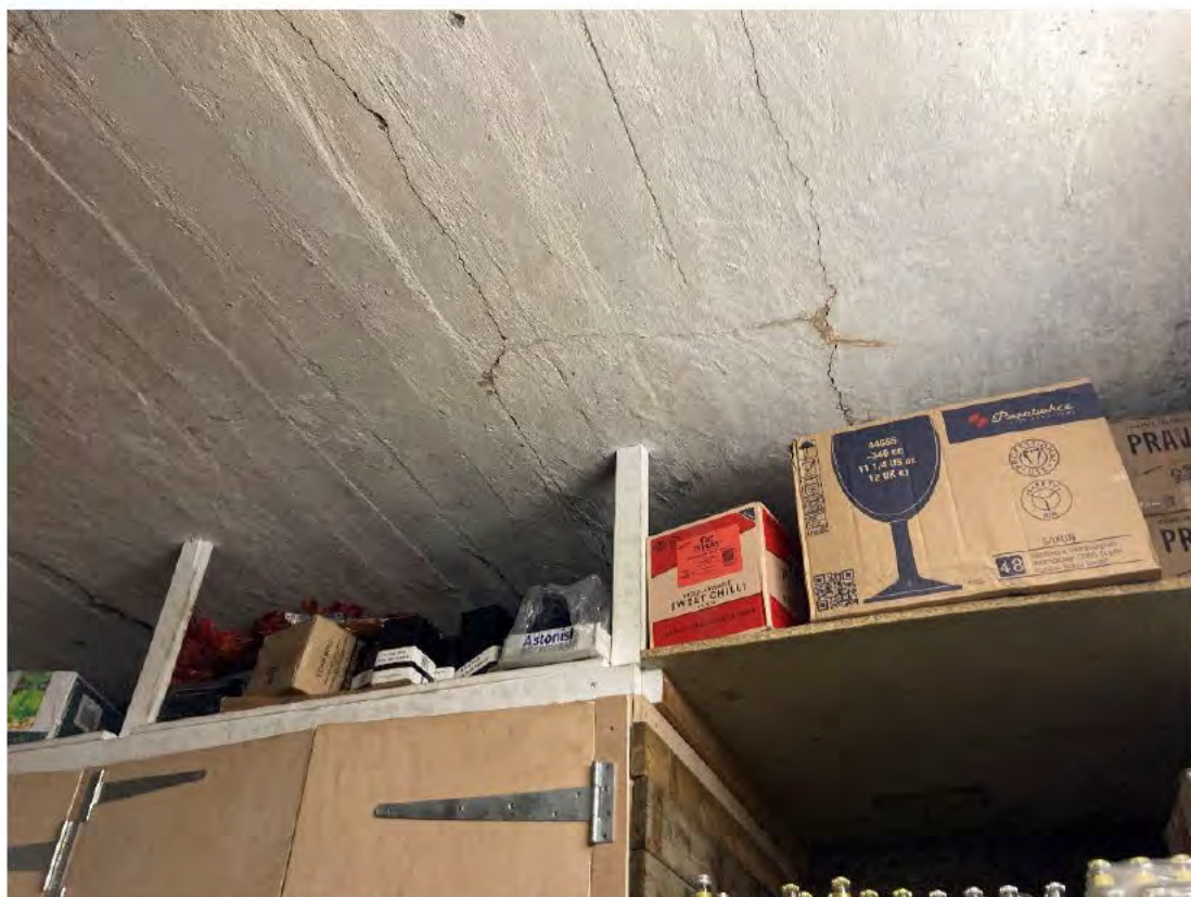
Photograph 12: Condition inside Arch No. 135. Deck soffit presents widespread cracking.
