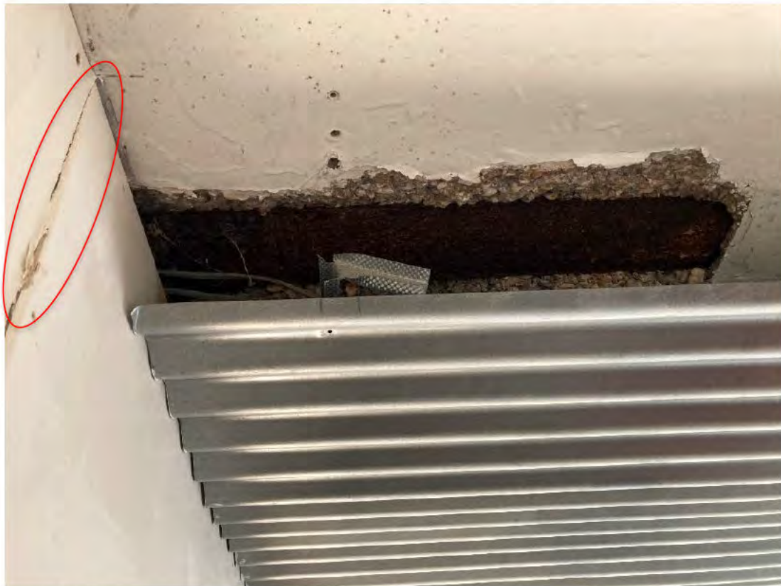
Photograph 9: Arch No. 134, Deck soffit presents honeycombing and rust staining above ceiling panel. Also note evidence of water dripping down the supporting wall.
